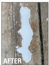
Once the repairs were made to the entrance of the warehouse, the floor was coated with **Eracoat 2K Rapid** Light Grey and broadcast with (Non Skid) NS150 aggregate. This was followed by a finishing coat of Eracoat 2K Rapid Light Grey.
